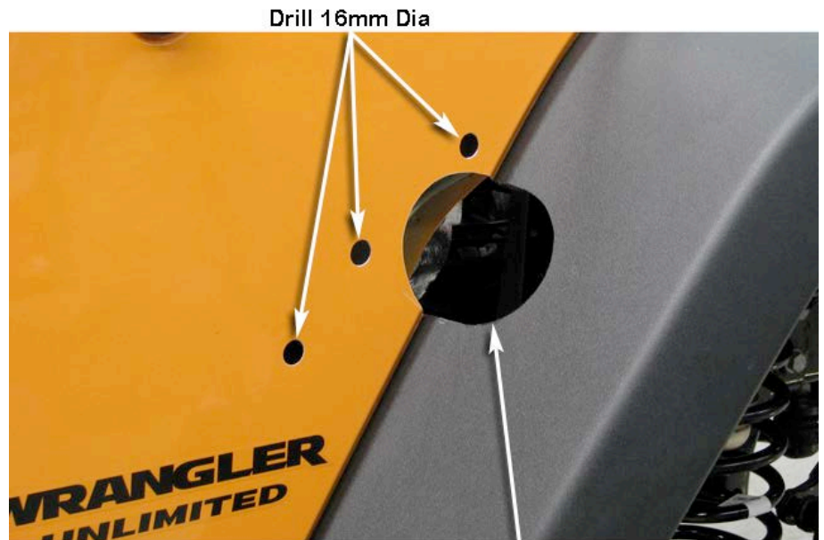
Cut Using Air Body Saw
